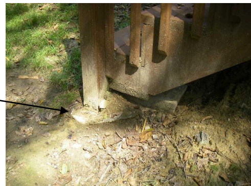
Sample – under eroded air conditioner pad
