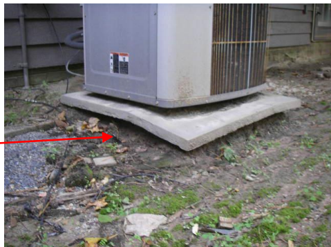
Sample – erosion Improperly supported unit
