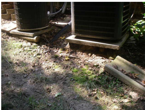
Sample – under eroded air conditioner pad
