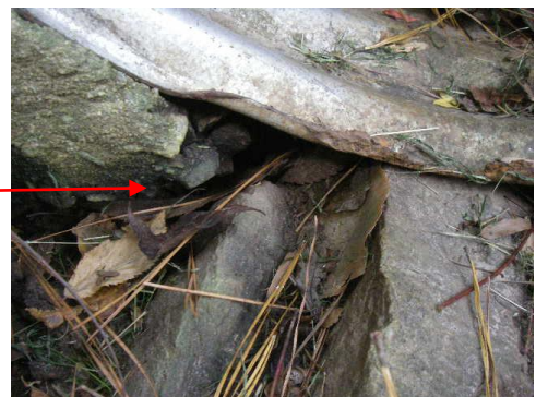
Water is running under culvert
