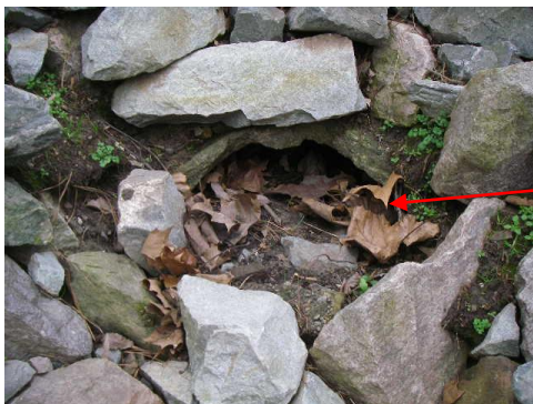
Culverts needing cleaning
