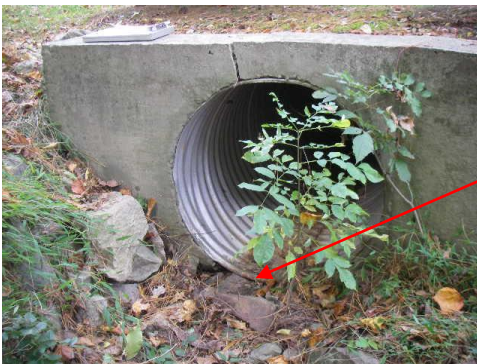
Water is running under culvert
