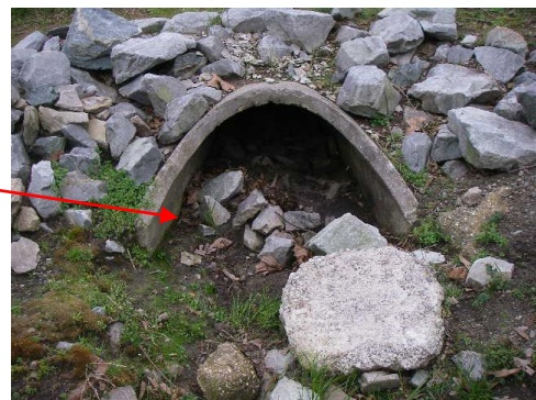
Culverts needing cleaning
